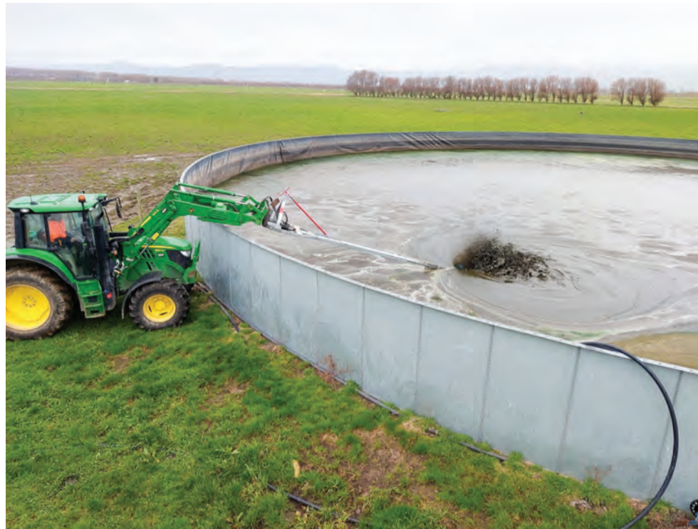
Above ground effluent tanks need a good stirrer to keep the effluent well mixed.
