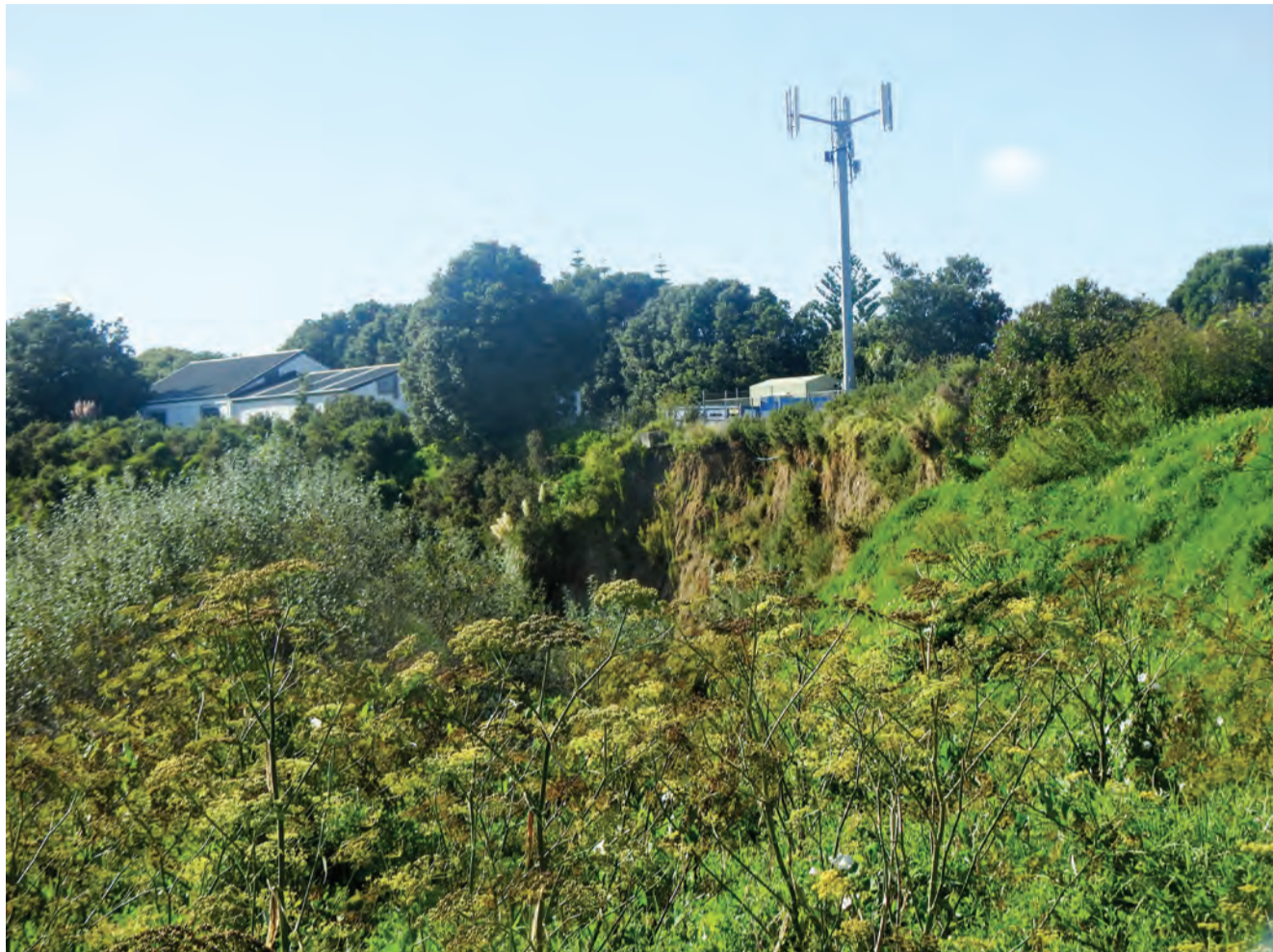
Something needs to be done about this eroding cliff.
