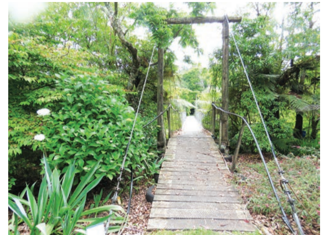
The swing bridge.
