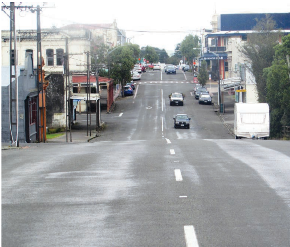
Bridge Street in Eltham. First in New Zealand.
